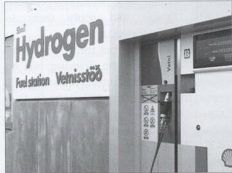
A hydrogen "filling station" in Iceland for fuel cell vehicles.
