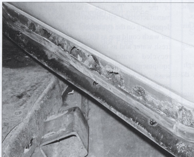
The close up view shows the extent of damage.
