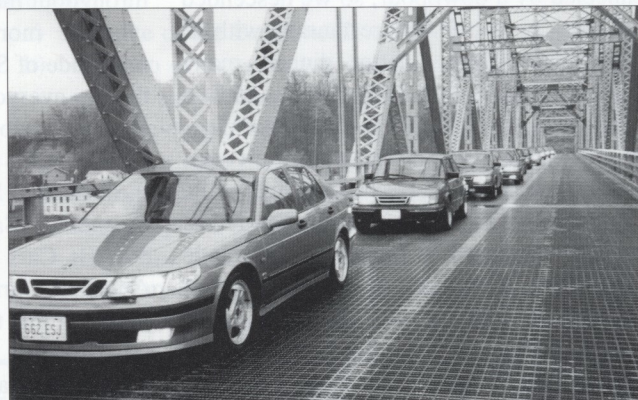
Crossing the Mississippi River at Mason, IA. Photograph by Paul Ellis
