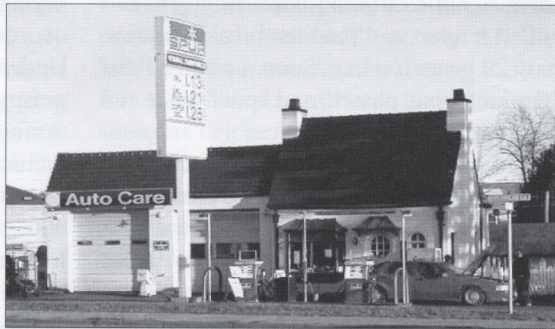
This full service station was built in the 1920s according to the "Pure Oil" design standard.
