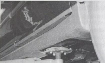
Figure 21: Recessed lower door sill, plastic cladding, and cladding on door bottom edge.
